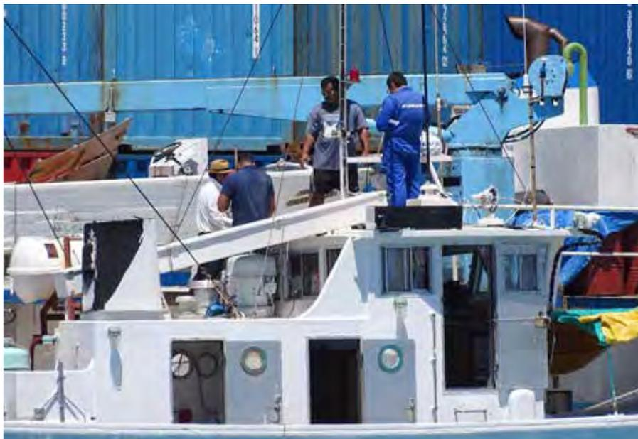
Figure 32: Fisheries mechanics and Furuno expert installing the new echo sounder on RV *Manauai*
