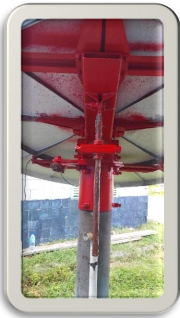
Figure 41: VSAT dish ongoing maintenance.
